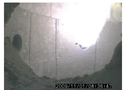
Calciner 6 burner nozzle
