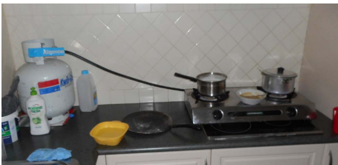
Wok type burner connected to LP Gas cylinder inside
