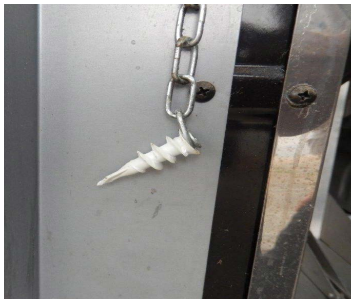
Inadequate restraints
