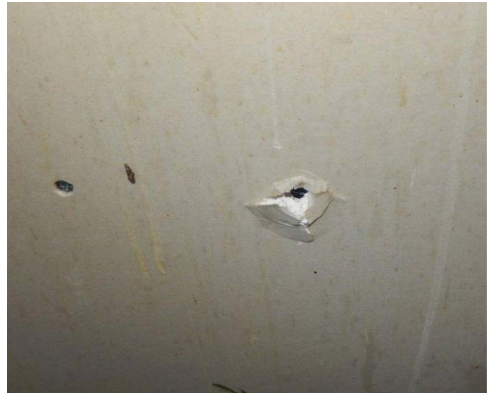
Damaged anchorage point
