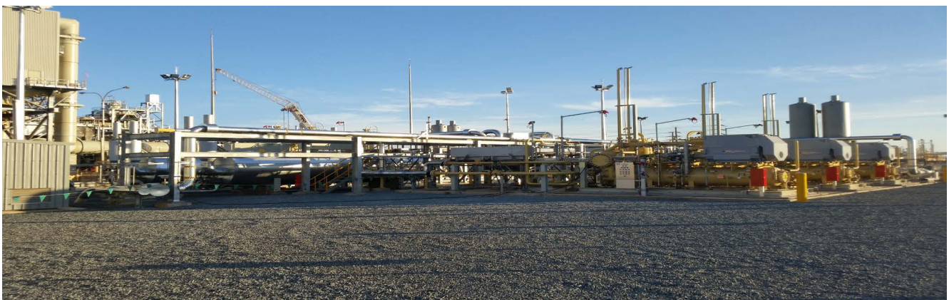
South Hedland Power Station under construction
