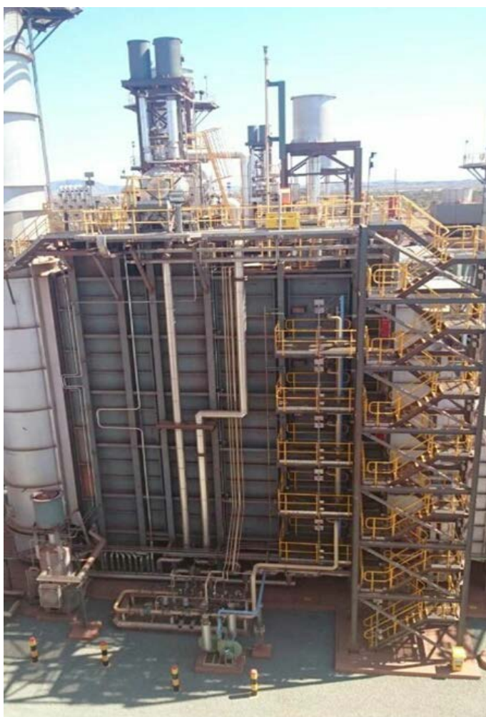
Yarnima Power Station Heat Recovery Steam Generator at Newman
