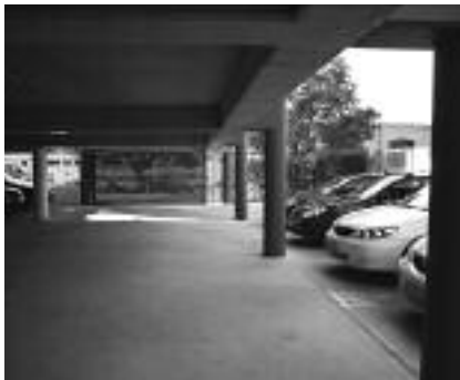
A car park with open sides. Consumer gas piping installed beneath the ground in this type of installation must comply with the requirements for 'piping beneath a building and in the ground'
